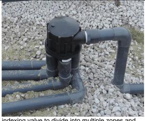
indexing valve to divide into multiple zones and feed sequentially by a single pump.
