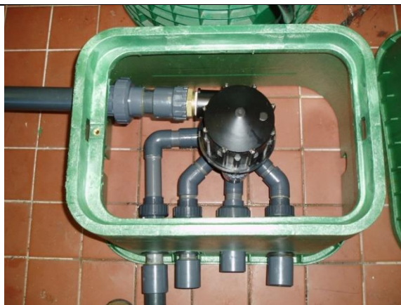
Example of a 4 zone pipe network using a 4 outlet indexing valve
