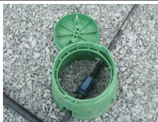
Our Indexing valves can pump water to 2- 6 independent cells in sequence using a single pump. Useful for large systems or to use small parcels of a small site.
