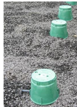
Orifice shields are available to prevent holes being blocked with soil –or cuts of 110 mm pipe can be placed directly over pipes.
