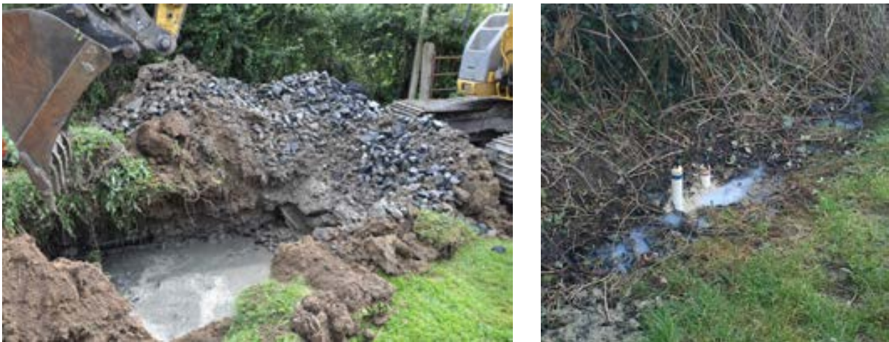
Figure 2.3. Site A soakaway being excavated and lysimeters in adjacent ditch.
