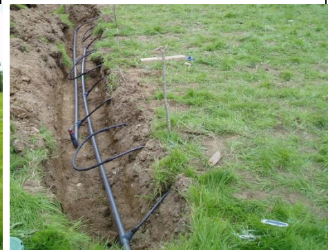
Driplines connected to manifolds in a single trench
