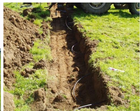
Driplines ready for connection to manifolds
