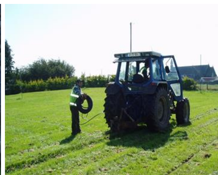
Mole ploughing of dripline into the hurling field using a farm tractor attachment
