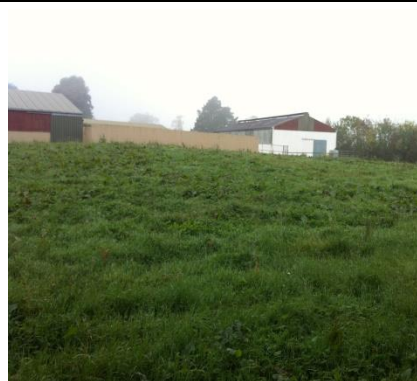
Dripfield operating satisfactorily 6 months after installation
