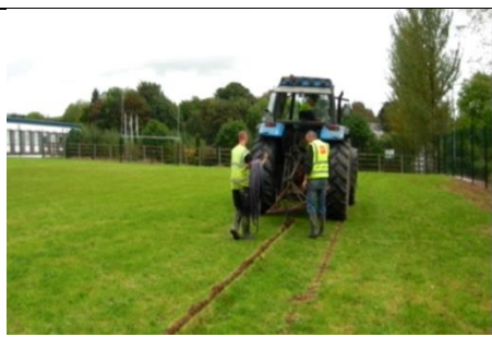
Mole ploughing of dripline into the playing field using a farm tractor attachment with little or no damage to the soil structure and no aggregate
